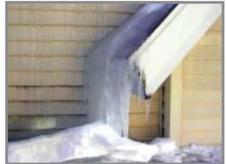
Typical Examples of Ice Dams
